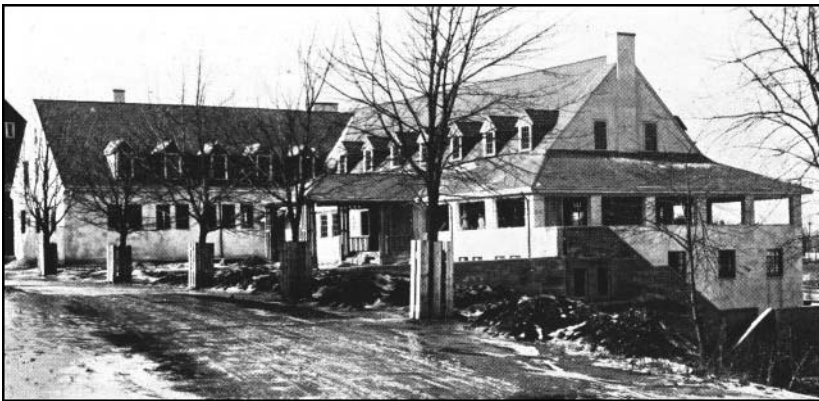
New home of The Commonwealth Country Club, Chestnut Hill, Mass., the interior of which has not been completed.
